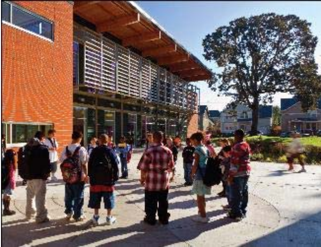
At the Rosa Parks School in Portland, Ore. students don't have to go far to get to the Boys and Girls Club of Portland, which is connected to the school building.
