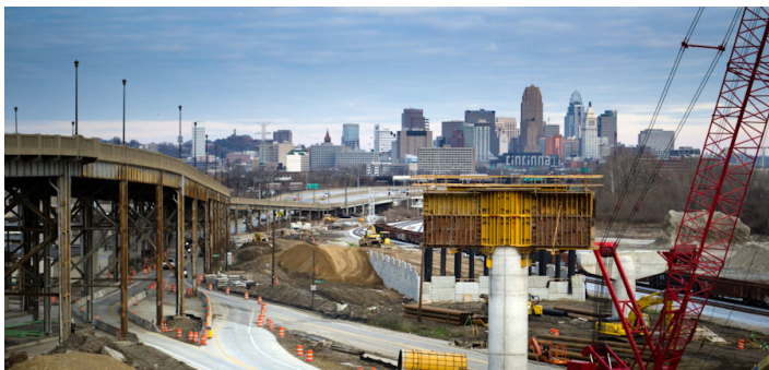
Waldvogel Viaduct Renovations. Photo from urbancincy.com
